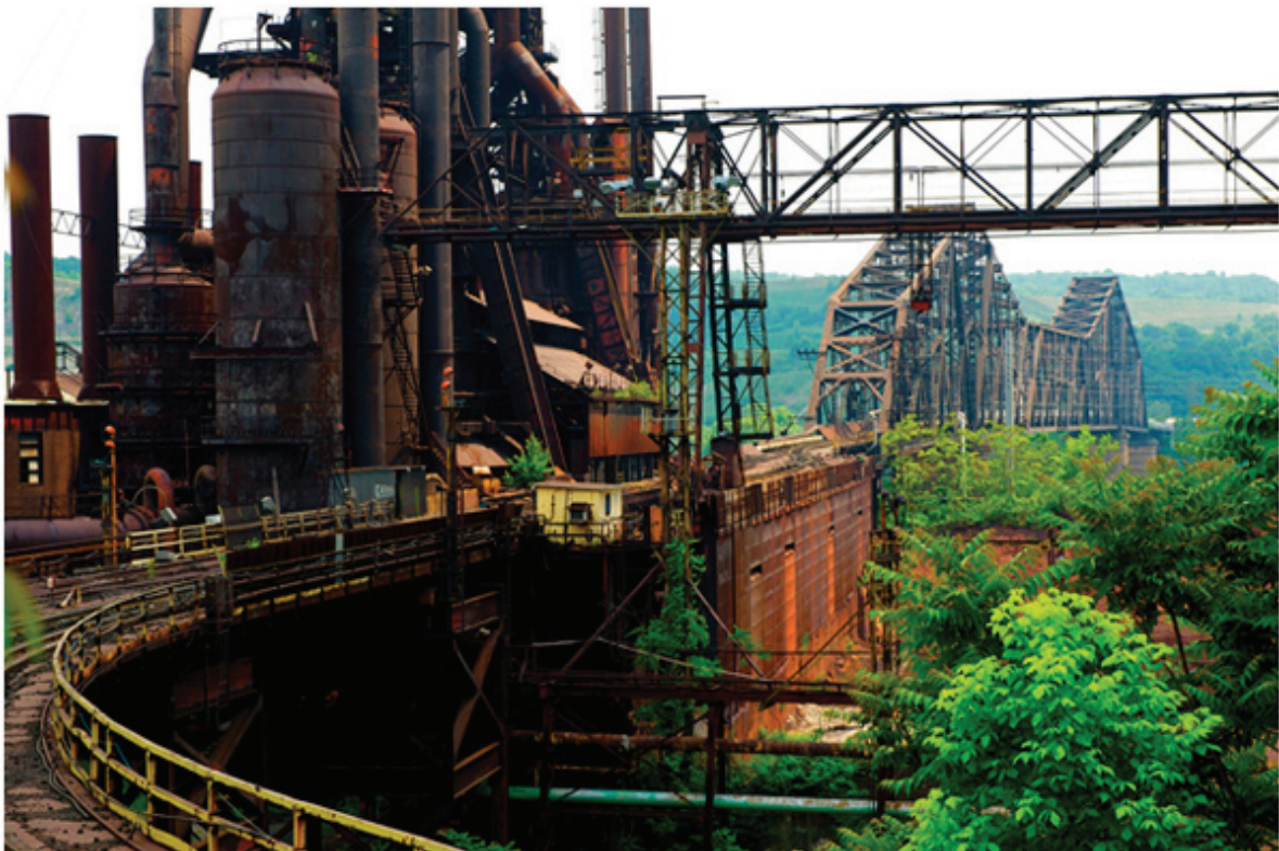
Fig. 4. Still mill in Stuebenville, Ohio. Источник: http://Dobrihomjachok.livejournal.com/29304html
